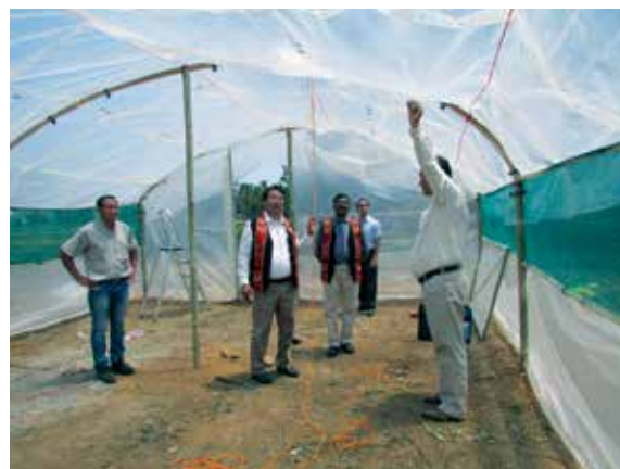
Construction of low cost polyhouse with bamboo frame at Peren, Nagaland
